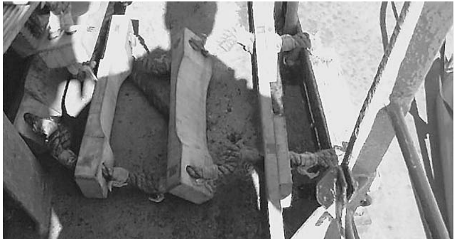
A replacement spreader used to wedge the ladder against the rails and the ropes pass over a sharp strake. If a pilot boat “hung up” on this ladder it would break at this point!
