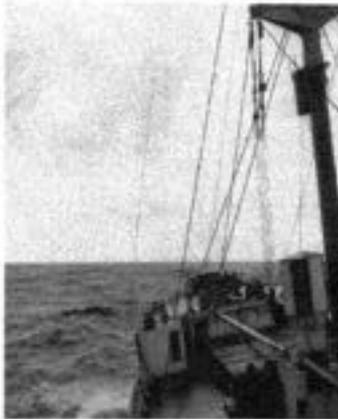
This picture was taken a few days before the storm and everything looks neat and tidy the deck cargo all stowed and lashed down, the derricks in place and the ventilator cowling beside mast intact. The anchor winch and the hand railing the fo'c'sle looking as it should.
